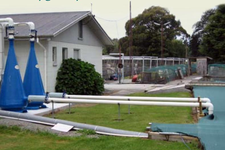
*Water from a nearby stream is pumped into the large blue cone-shaped towers called diffusers (right) where oxygen is added if required. The oxygenated water is then piped into the raceway. [Photo: Mark Crump, NIWA]*
