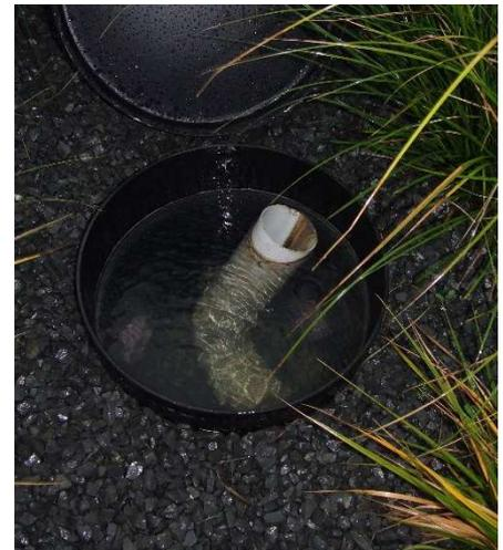
Figure 5: Discharge from the outlet of the greywater treatment wetland before it goes through the harakeke infiltration trench.
