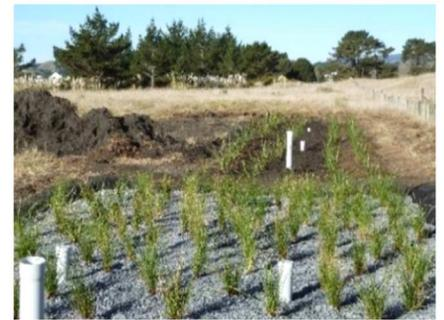
Figure 2: Constructing the greywater treatment wetland.
