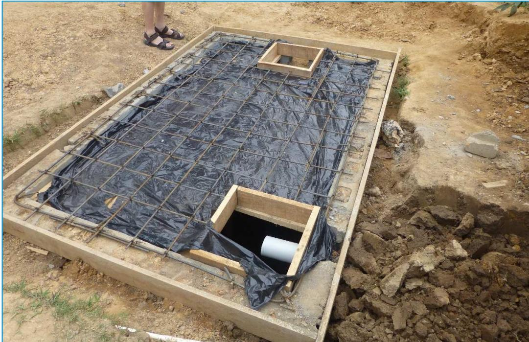
Figure 7: Completed household blackwater septic tank for 6-8 people. Dosing chamber and land application system vents are visible on far side of tank.
