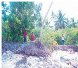
Coastal erosion, Kiribati 2004. Photo courtesy of Mineral Unit, Kiribati
