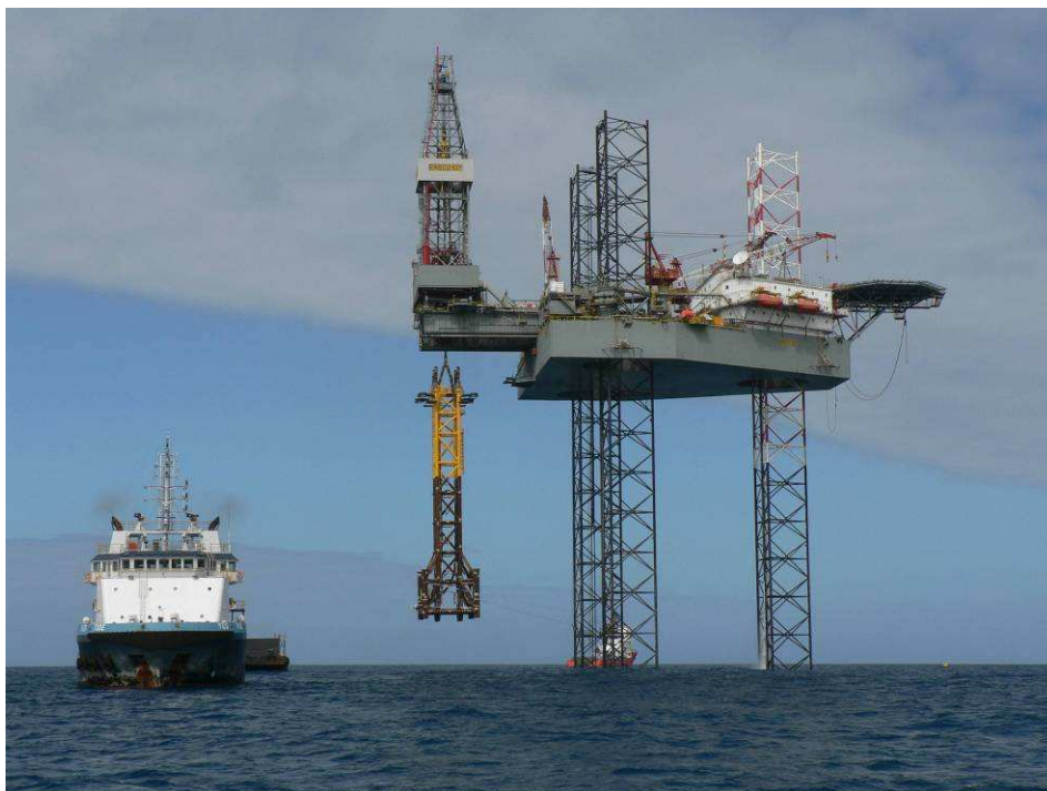
Figure 4.2.15 – The “jack-up” used for the Kupe development, lowering the wellhead platform jacket
