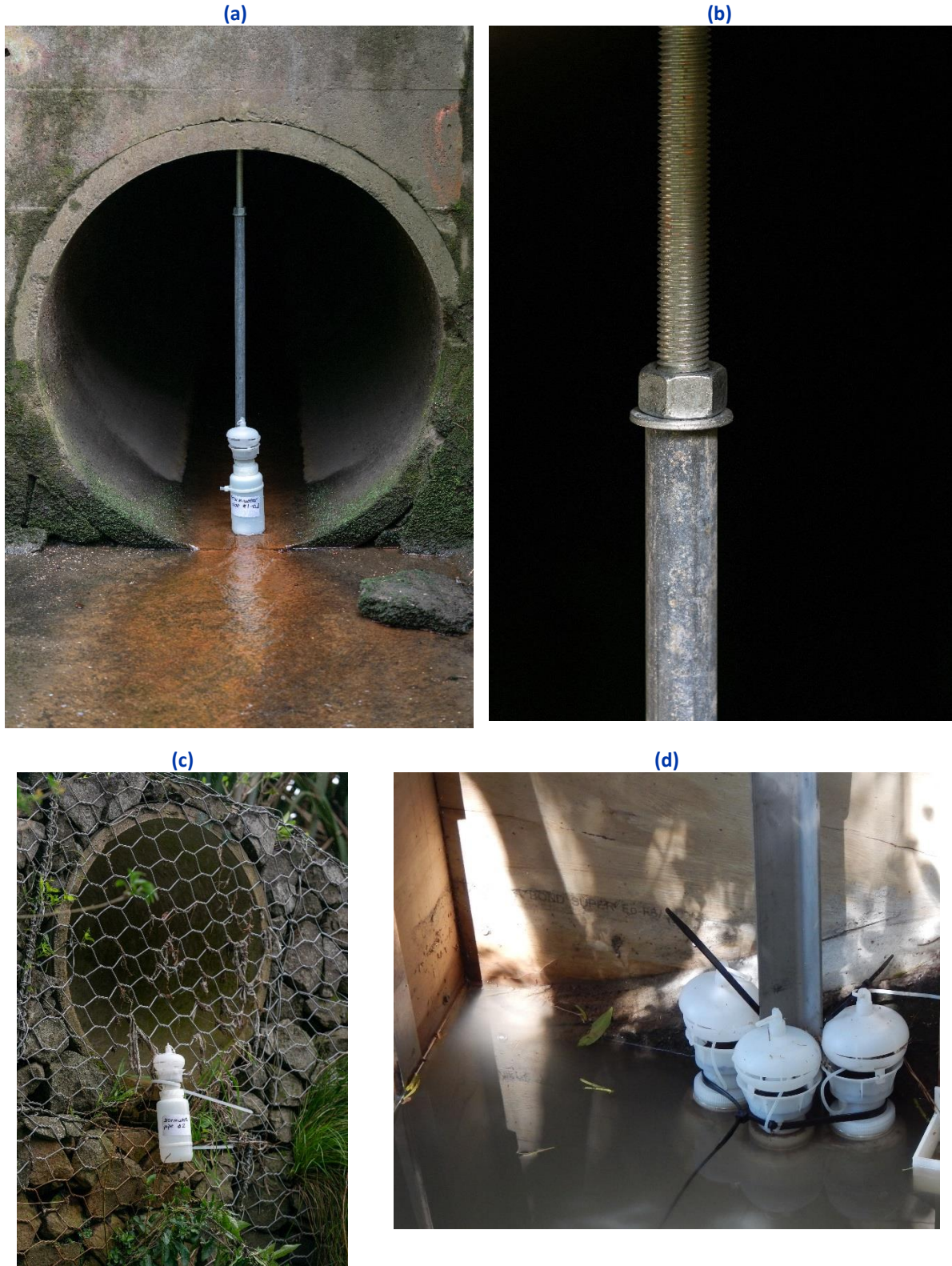
Figure 6: Bottles mounted (a) with an extendable threaded rod; (b) close up of the threaded rod; (c) using existing steel mesh on a stormwater outlet; and (d) to a piece of steel angle, dynabolted to the side of a stormwater outlet wingwall.
