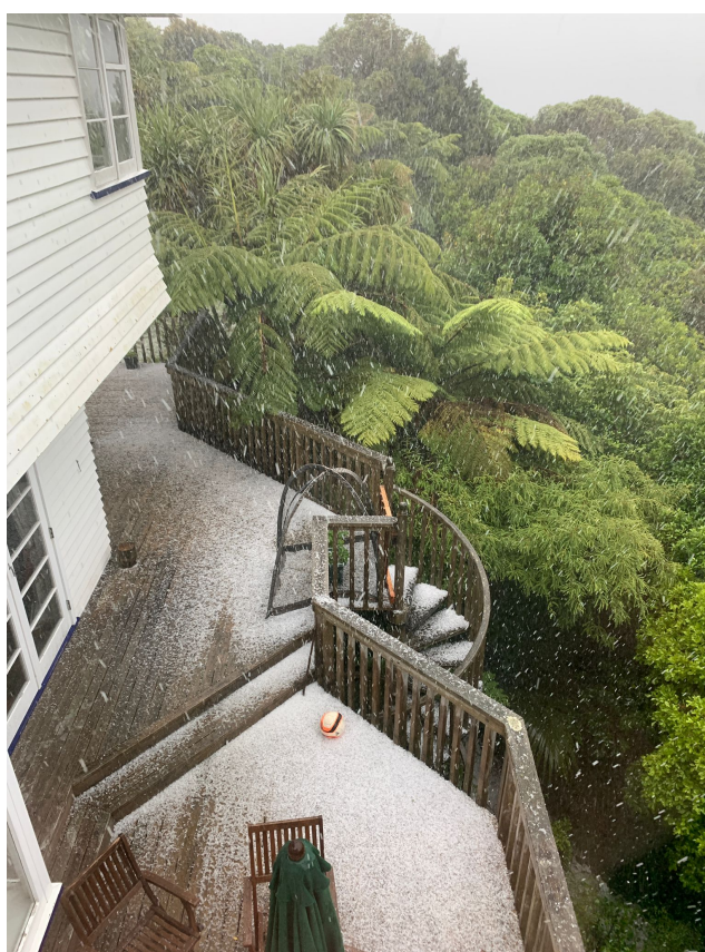
Photo 1: Hail in Wellington on 12 December. Widespread hail was reported across the hill suburbs, while wind damage occurred in the Hutt Valley.
