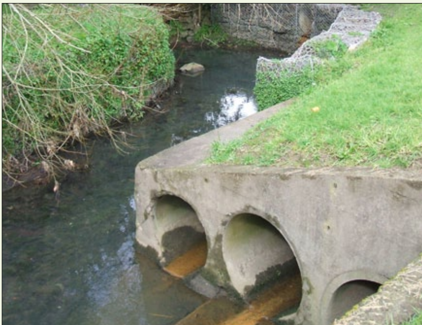
A combined sewer overflow outlet on Meola Creek, Auckland, during dry weather. Overflows of raw sewage are common following heavy rainfall and have contributed to the downstream degradation of both the creek and tidal inlet habitats (J. Gadd, NIWA, 2011)
