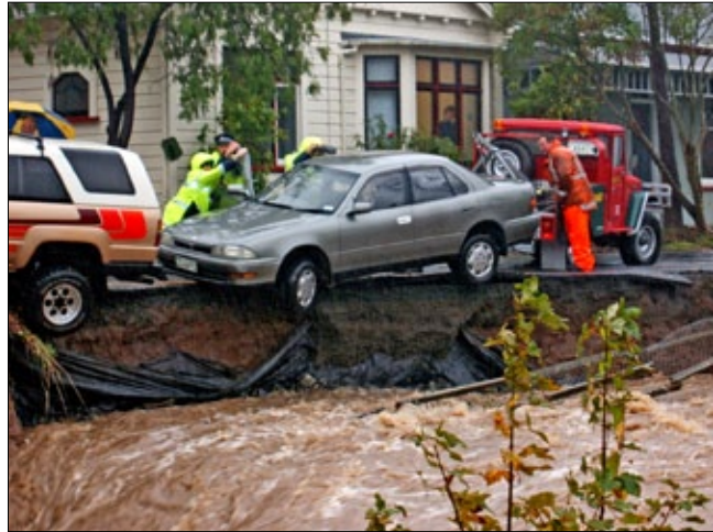
Flood erosion on the banks of the River Leith, Dunedin (A.J. Nancey, 2006)
