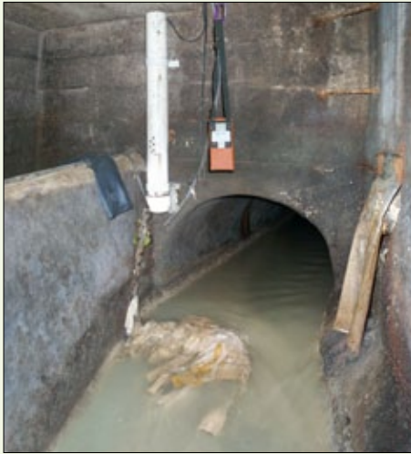
Combined sewer overflow in Auckland showing dry weather flow. The side weir is designed to be overtopped during heavy rainfall causing release of untreated wastewater to the receiving environment (P. Pattinson, NIWA, 2003)
