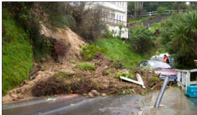
Slip in Devon St, Aro Valley, Wellington following heavy rainfall (Erika Mackay, NIWA)
