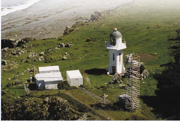
Baring Head Atmospheric Research Station and nearby Baring Head lighthouse.
