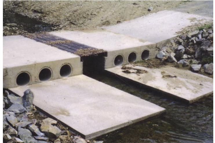
Fish-friendly ford design with an unobstructed channel in the centre.
