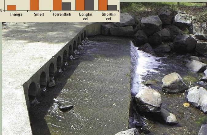
Ford on the Tapapakanga Stream, only 3 km inland from the sea. Note the shallow water over the apron and vertical drop at the end of the apron. The graph shows that this ford affects the passage of inanga, smelt, and torrentfish, but not eels.
