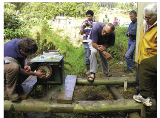
Renewable energy at Waipoua.
