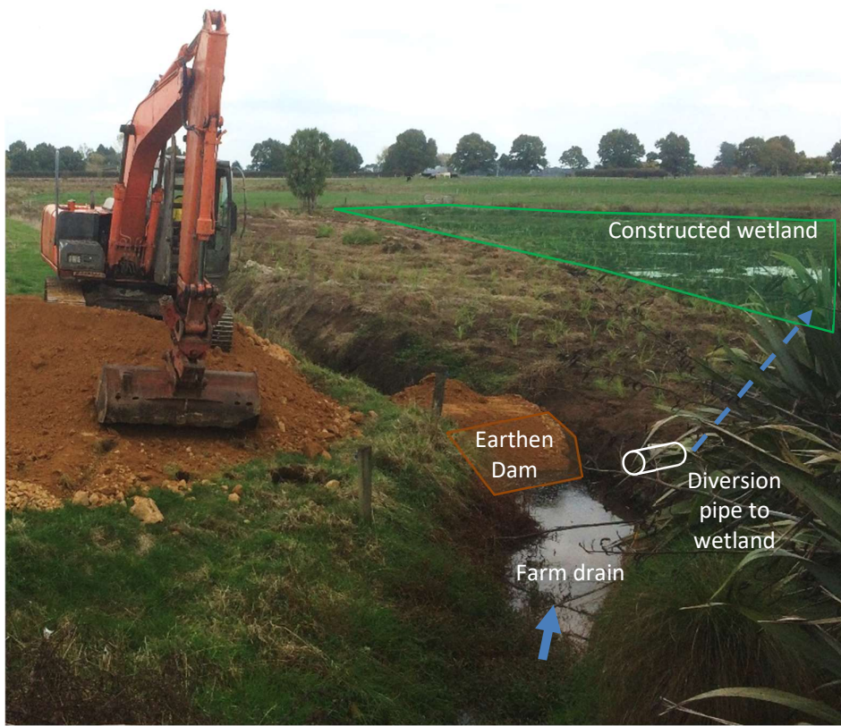
Figure 4: An off-stream wetland (in background) being connected to flow from a drain. An earthen dam (to be armoured with geotextile) has been constructed to block the existing drain. A pipe will be installed to divert the impounded water to the constructed wetland. Another pipe will be installed further downstream to feed this water back to the drain after passage through the wetland. Excess storm flows can still flow over the dam and down the drain.
