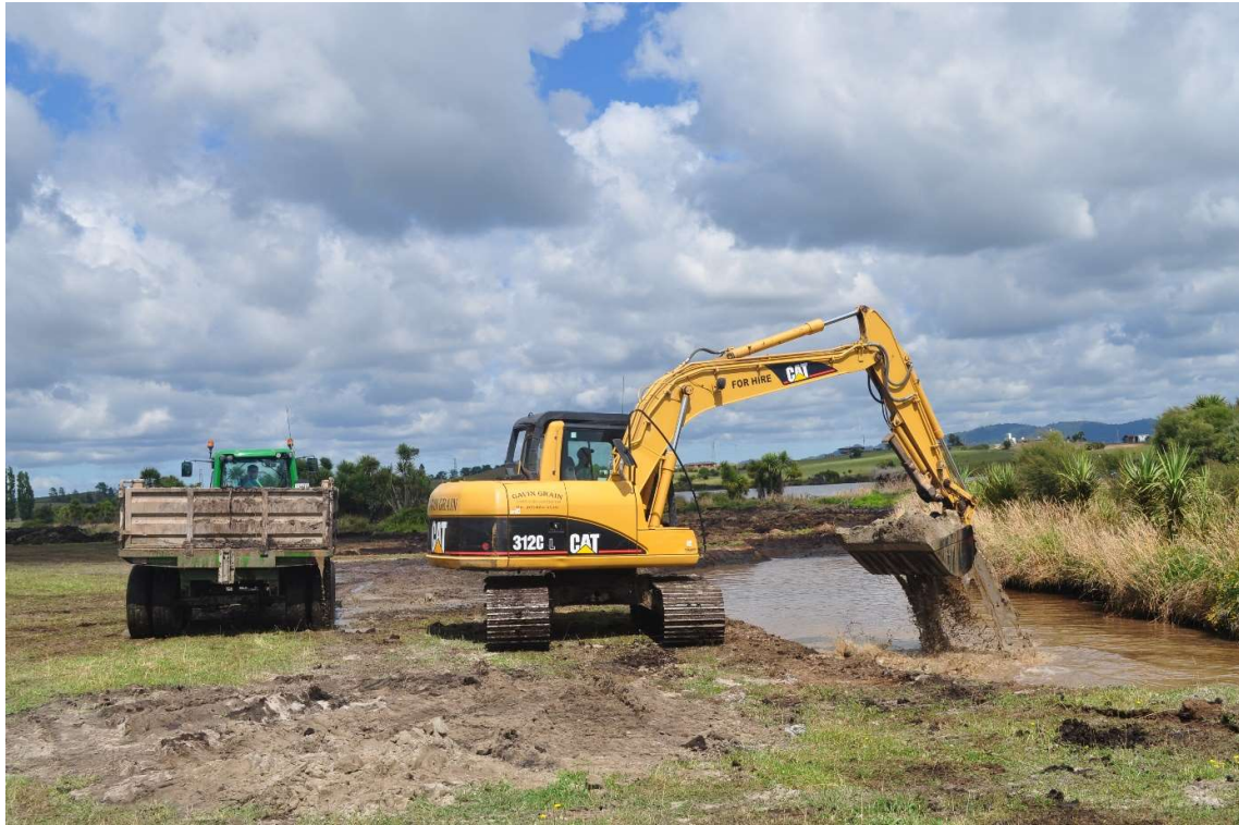
Figure 22: Emptying a sedimentation pond.
