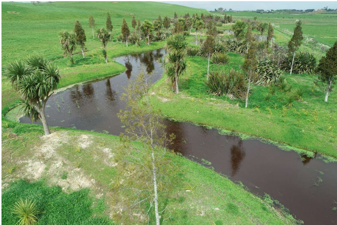
Figure 15: A wetland constructed in a retired area of restored native bush. The curved shape winding between the trees gives a more natural appearance. (Wetland plants are just becoming established).
