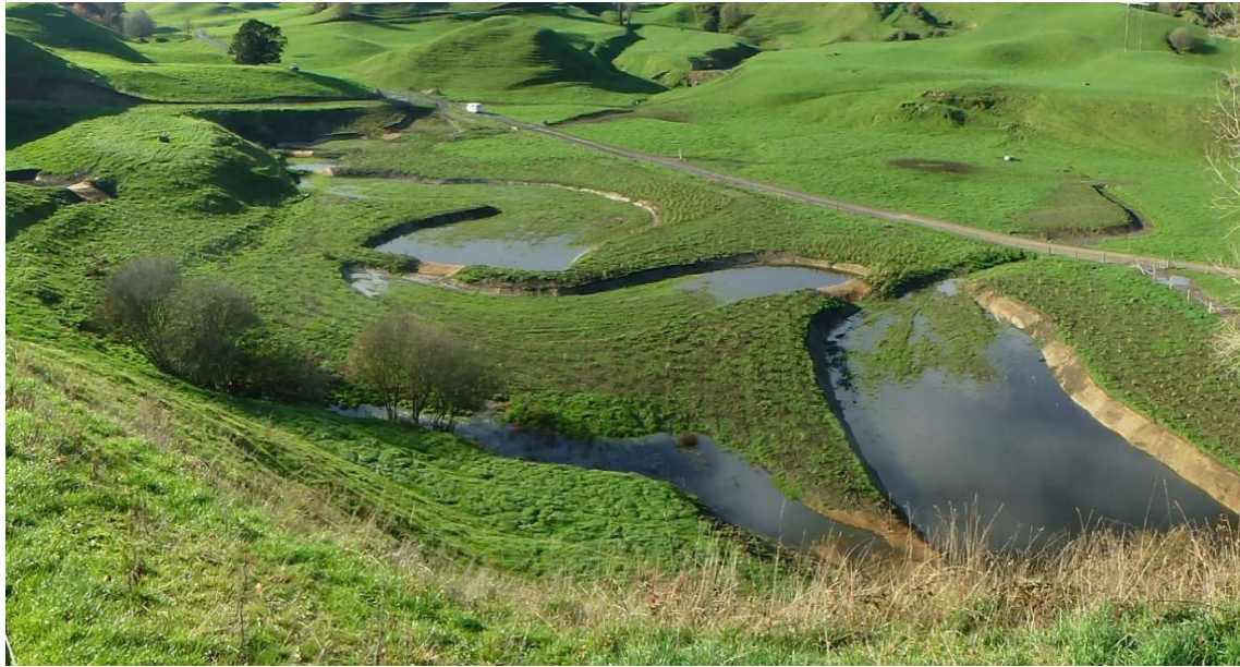
Figure 13: Example of a multi-cell wetland prior to planting. By creating multiple cells with a serpentine design, the bund height between cells is kept to a minimum. The design allows treatment of three major drain/stream inputs as well as runoff from the raceways. Use of curved edges to the wetland cells creates a natural appearance. Note also Figure 14.
