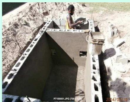
Construction of septic tank. (See KoroSan #2-5)
