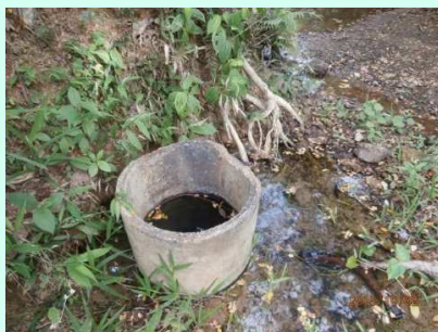
This is an emergency water source (a spring) for the village but it is not properly protected or covered.
