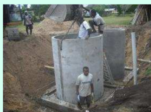
Excavating for black water collection and pump chamber
