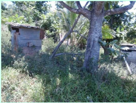
The toilets are located on higher ground whilst the borehole is situated below. There is the risk of faecal contamination from the toilet.
