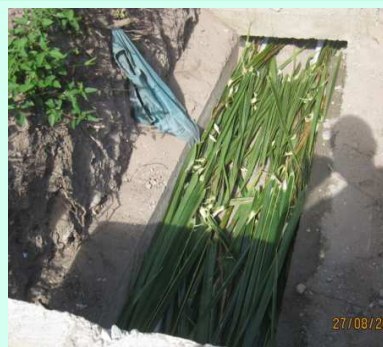
LAS system on sandy soil. (See KoroSan #2-5)
