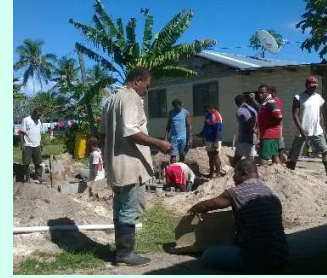
Digging land application trenches
