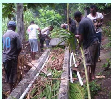
Construction and completed above-ground waste-water treatment systems for low permeability, high water table clay soils.
