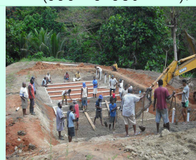
Constructing wetland for black water treatment behind village
