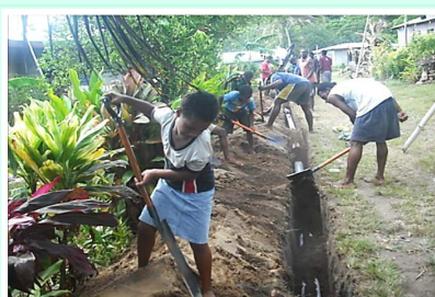
Digging trench for new water reticulation system around village
