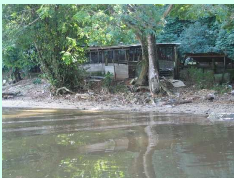
Piggery waste draining to river.
