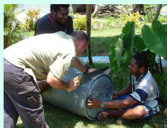
Preparing drums for household grey water infiltration (see KoroSan #7).
