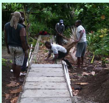
Construction and completed above-ground waste-water treatment systems for low permeability, high water table clay soils.
