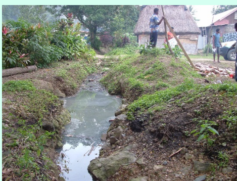
Wastewater ponding in a drain flowing into river.
