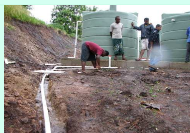
Installing drinking water tanks to remove sediment and provide storage
