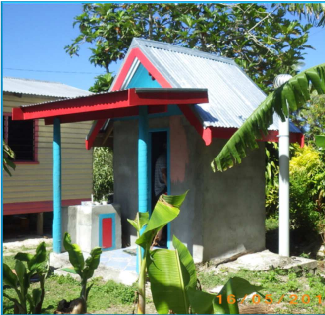
Figure 3: Two different ecoVIP2 toilet building designs. Note provision of hand washing facilities outside the toilet on the left, with drainage directed well away from the pit.
