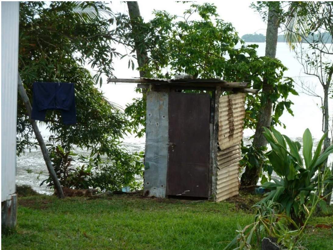
Figure 12: An unsuitable site for a pit toilet. Good views, but a high chance of contaminating the lagoon and being damaged during storms.
